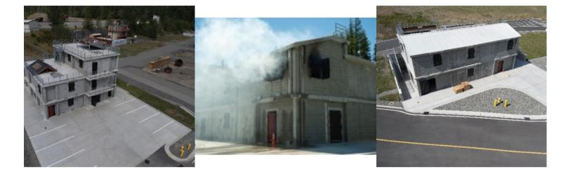
The Fire Training Academy's new burn buildings are open for training! The buildings are comprised of an Apartment-Style Burn Building, which includes three stories, five burn pits, and ventilation props on the roof; and a Residential-Style Burn Building with one story, a daylight basement, three burn pits, and a Fire Control I/Burn to Learn Room.
