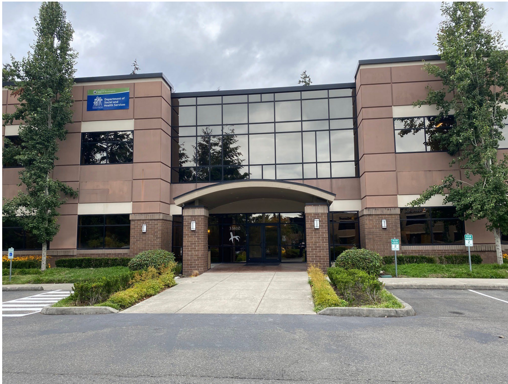
Federal Way Tox Lab – North Building Entrance
