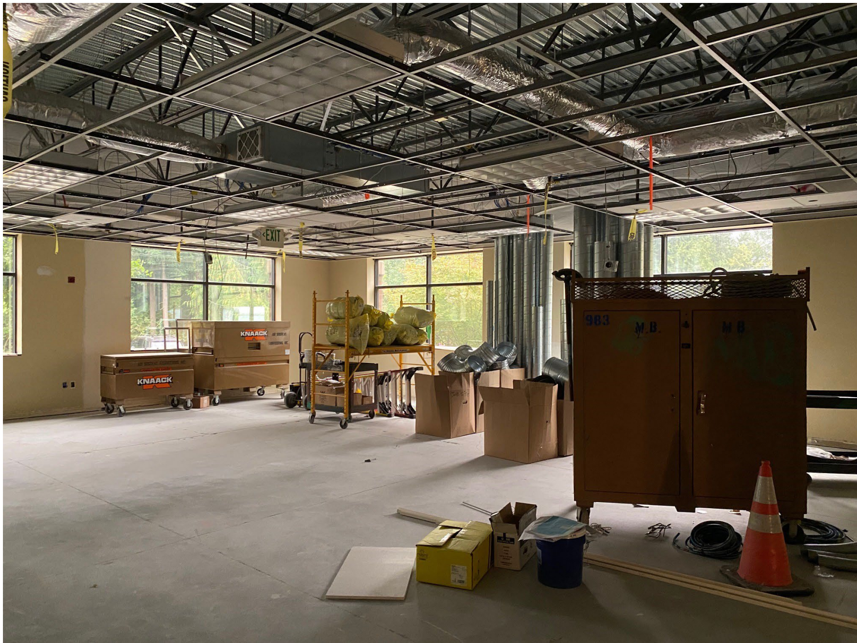
Federal Way Tox Lab – Main Open Office
