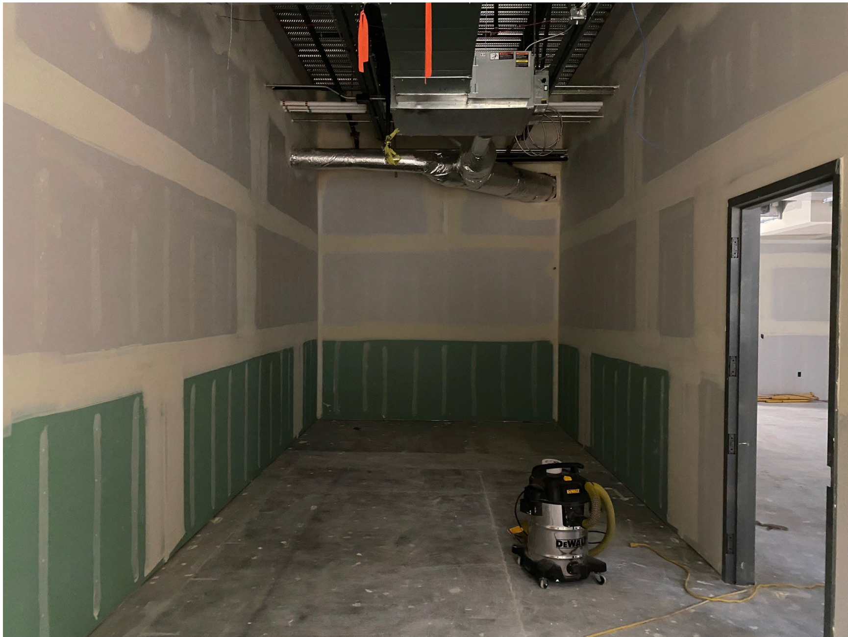
Federal Way Tox Lab – Evidence Walk-in Refrigerator Space
